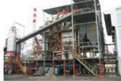
Biomass power plant in Chainat province has used rice husk as a fuel with the potential capacity of 6.0 MWe.
