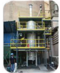
Biomass power plant in Chainat province has used rice husk as a fuel with the potential capacity of 6.0 MWe.
